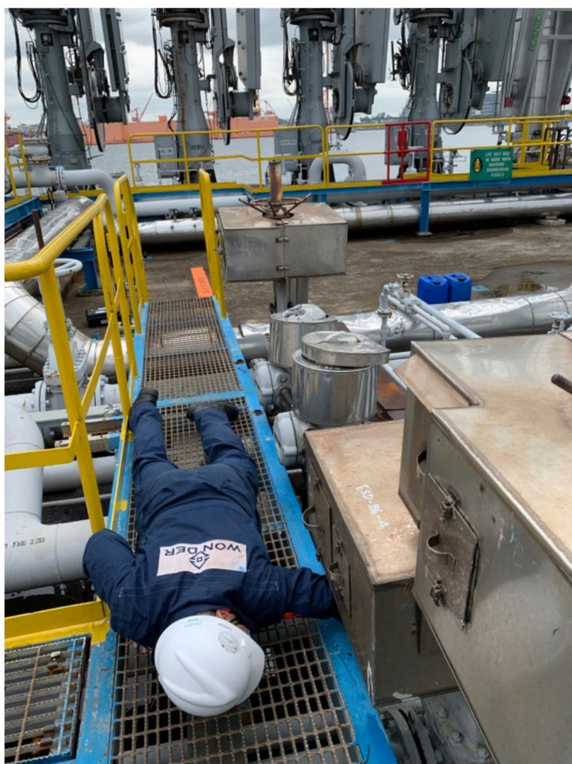
Figure 2. Conventional MOV replacement site survey.
